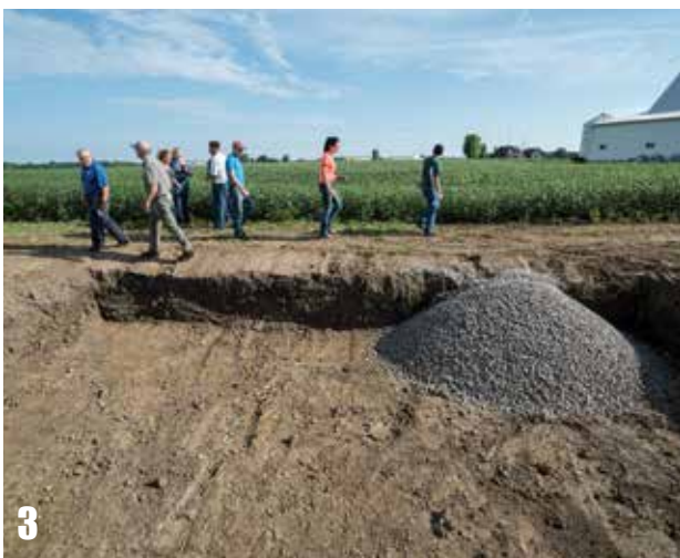
1. Area agricultural professionals get an up-close look at a sub-surface nutrient placement toolbar at Kellogg Farms. 2. Kevin King from USDA-ARS discusses how edge-of-field monitoring equipment takes water samples for later testing. 3. A blind inlet phosphorus filter bed being constructed on Kurt Farms. 4. Surface water flume for collecting samples for edge-of-field monitoring.
