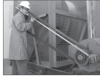
Using a straight edge to check alignment
