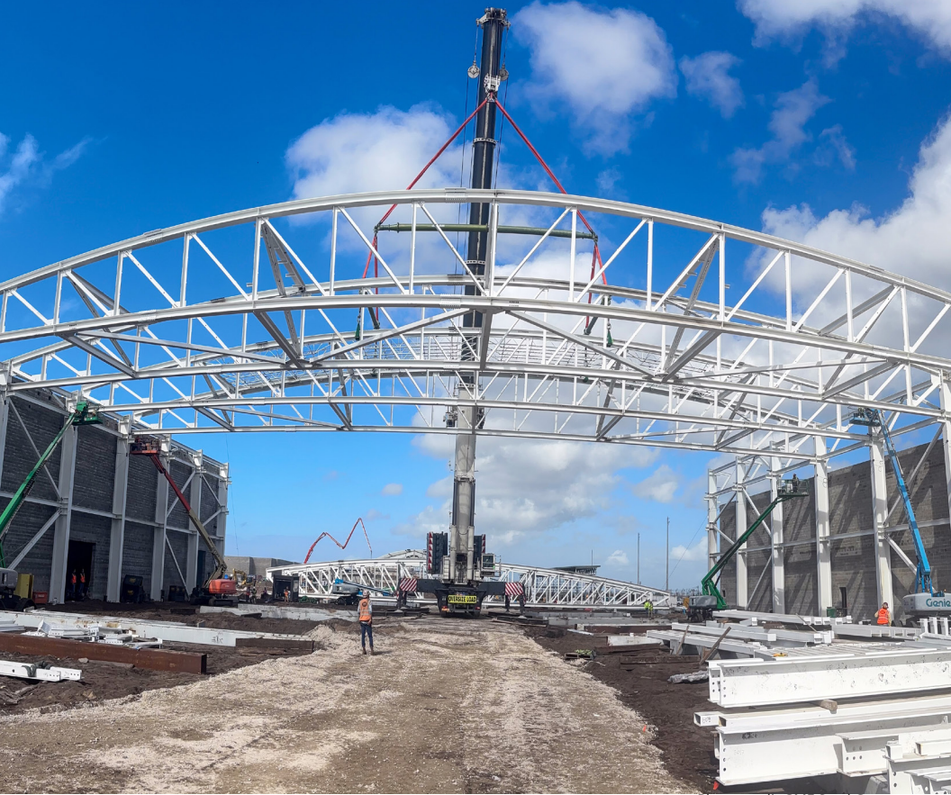
Photo credit GMF Steel Group
