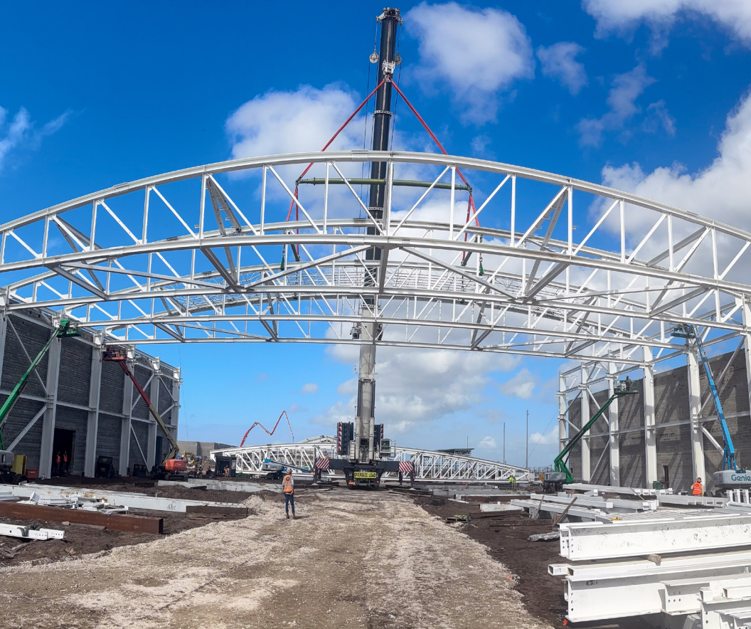
Photo credit GMF Steel Group
